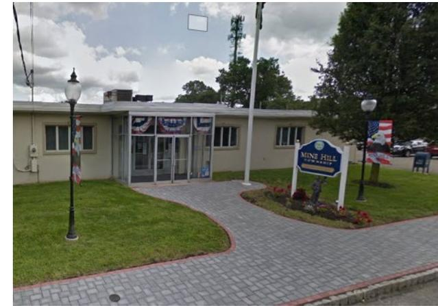
A rain garden can be installed in the turfgrass area near the building to capture, treat, and infiltrate rooftop runoff. A preliminary soil assessment suggests that more soil testing would be required before determining the soil's suitability for green infrastructure.
